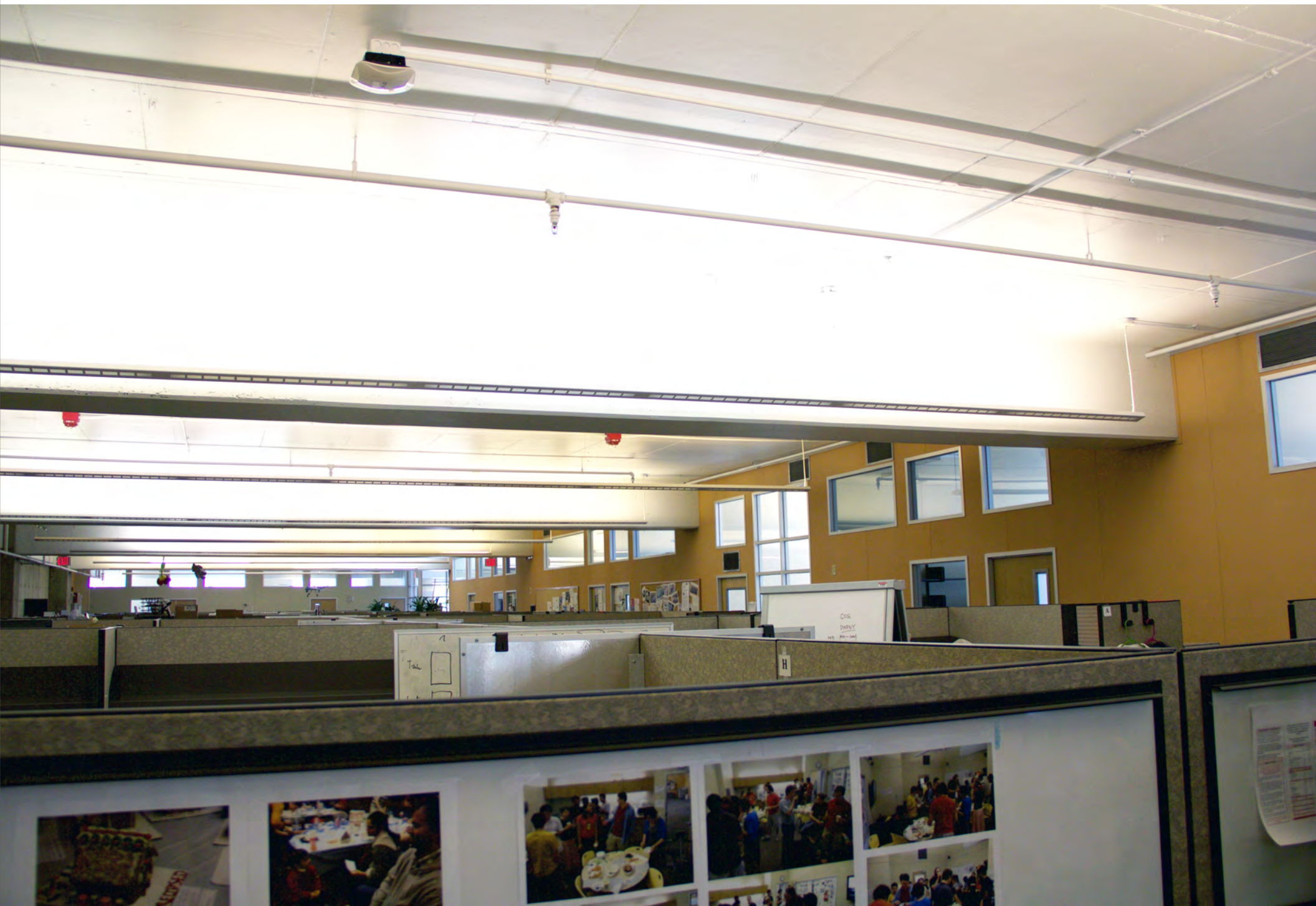
7. Faculty Offices Wall
