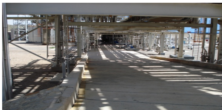
Figure 1. A view of pipe supporting structure
